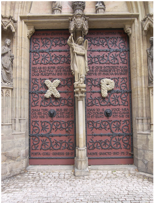
Figure 17. Erfurt, cathedral – wrought iron is applied as surface decoration only (without real fastening or suspension role)
