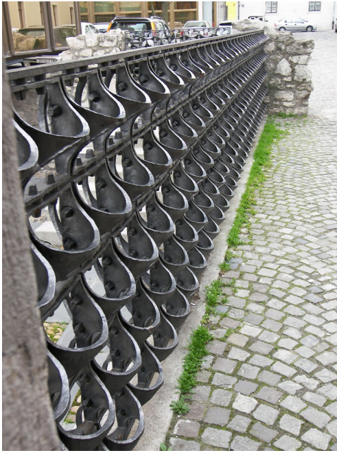
Figure 13. Budapest, Castle of Buda – modern wrought iron railing – harnessing the versatility of the homogenous material regarding the shaping
