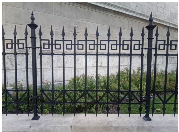
Figure 7. Museum of Fine Arts, Budapest. – A wrought iron fence poles shaped as spears
