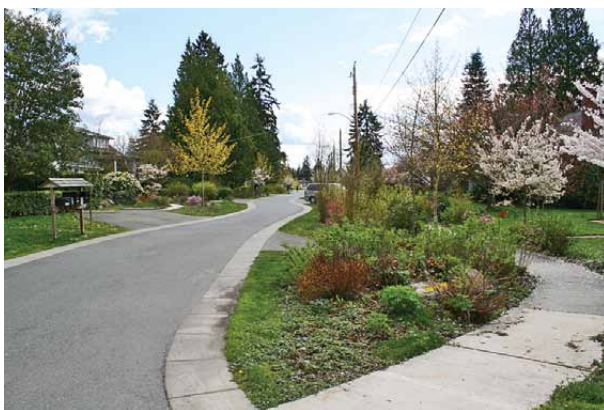
Fig. 4. Low Impact Design practice example (rain garden) in Seattle (USA)
