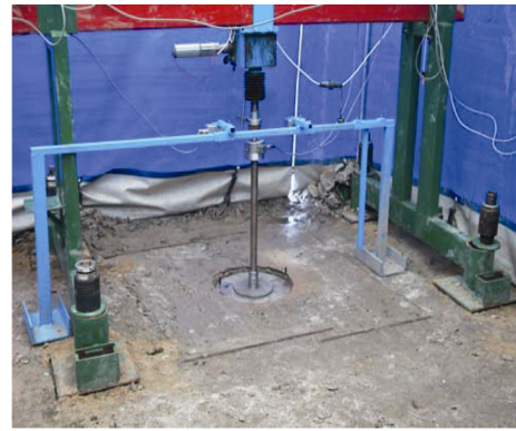
Fig. 7. Bucket load test device used for performing vertical load tests
