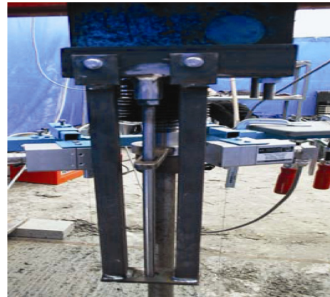
Fig. 8. Hanger bar reinforcement for vertical load tests
