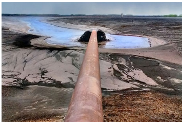
Fig. 3. The look of fly ash and slag landfill and devastated environment (the pipeline length is approximately 6.5 km from the thermal power plant Kostolac to the ash pond)
